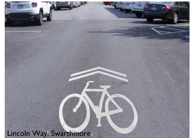
The most common bicycle lane is a striped section of roadway located to the right of moving traffic (left). When the roadway conditions provide enough space, bicycle lanes should be buffered from moving vehicular traffic (top). “Sharrows,” which are markers painted on the roadway to delineate where people should cycle, can be used on narrow roadways or streets that have a low volume of traffic (above).
